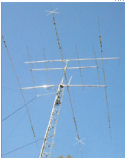
The antennas at WK4P. The tribander and wire did all the work this time.
